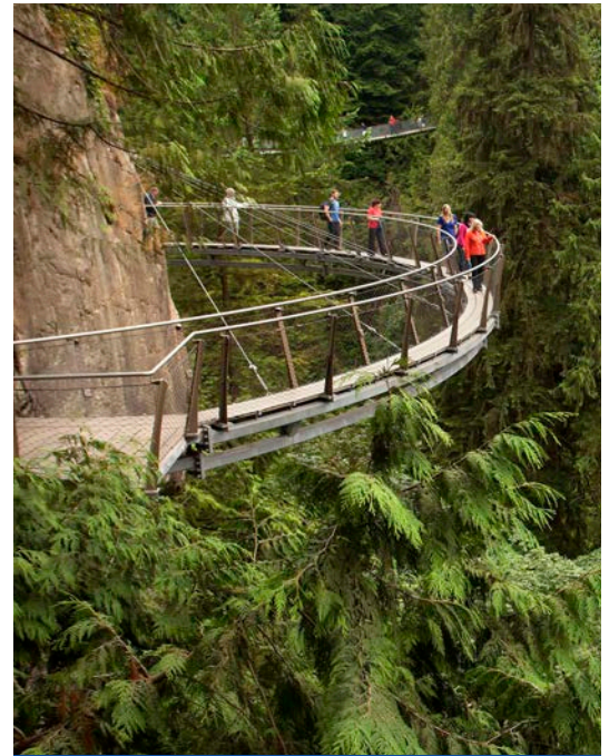
Capilano Suspension Bridge
